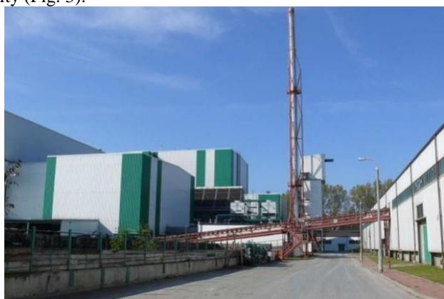
Fig. 3. Waste disposal plant in Warsaw (source: press release)
